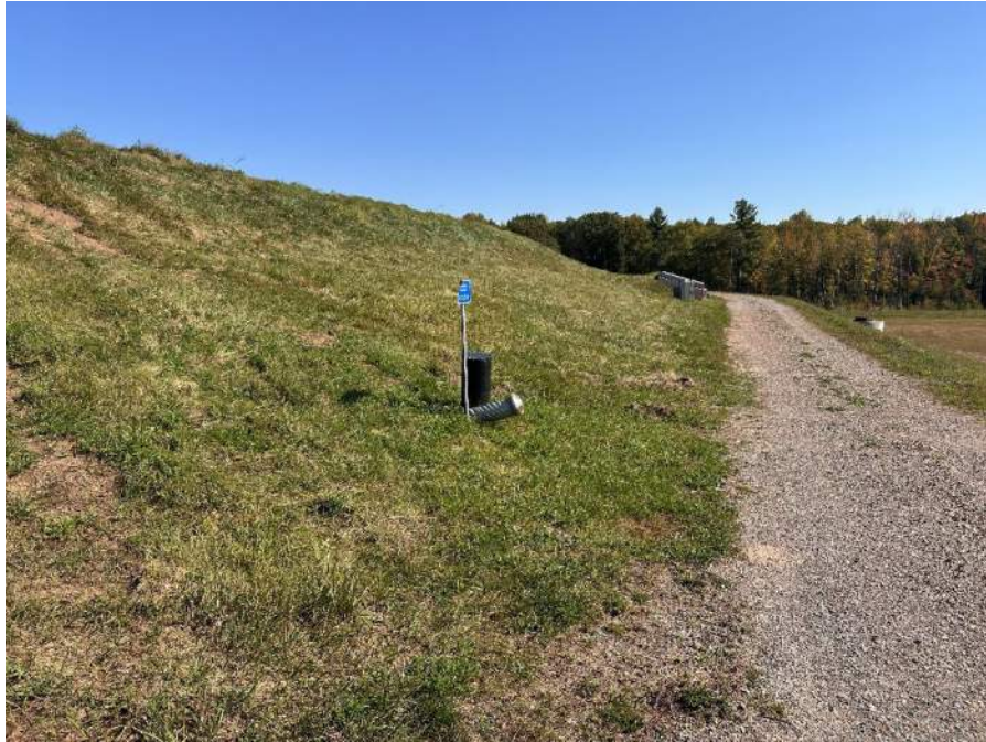
Photo No. 13 – Cell 2 south diversion berm and headwell pipe.
