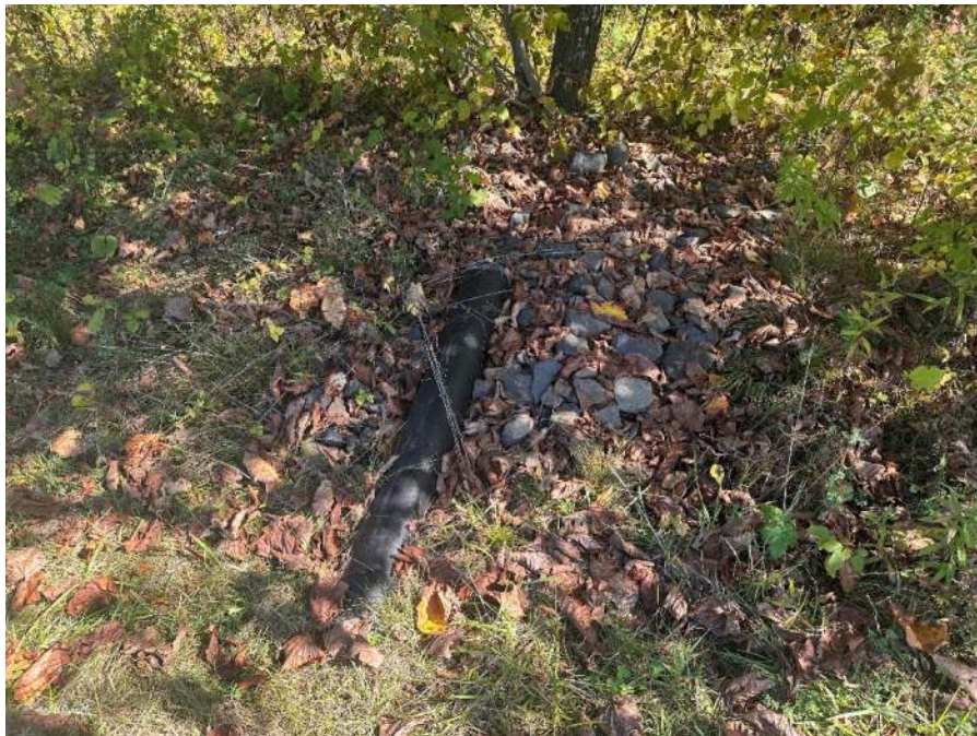
Photo No. 16 – Cell 1 gradient control outlet pipe.
