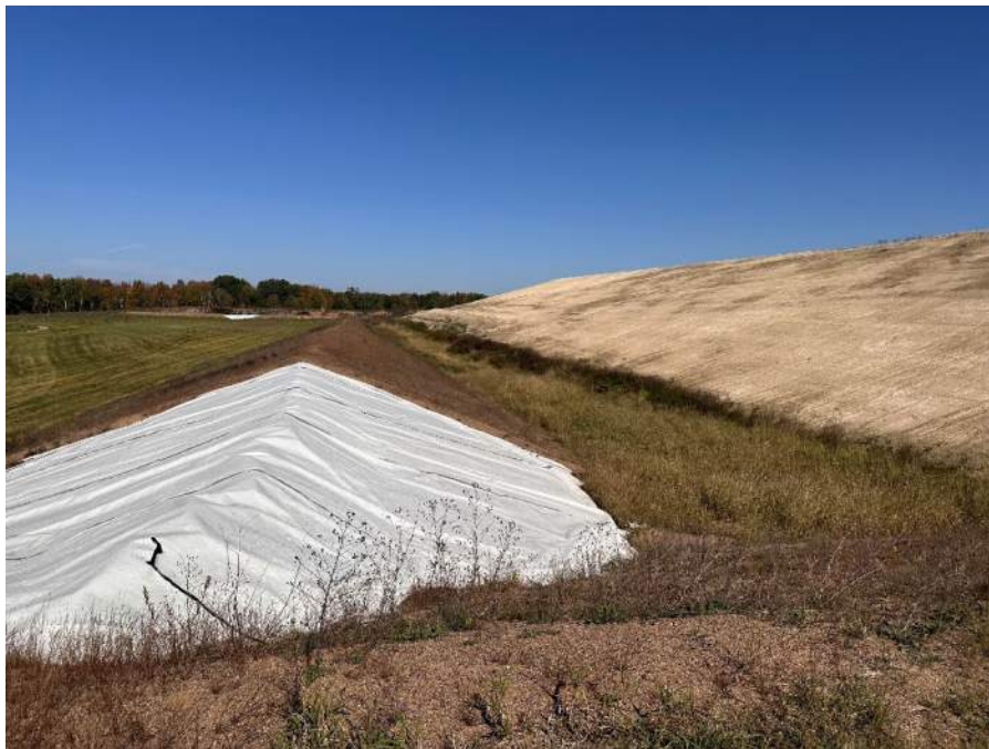
Photo No. 2 – Cell 2/3 intercell berm and leachate collection ditch along west side of Cell 2.
