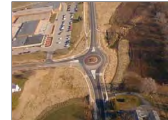
Lineville/ Rockwell roundabout in Howard
