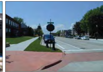
Curb extension along Grant Street in De Pere, Wisconsin
