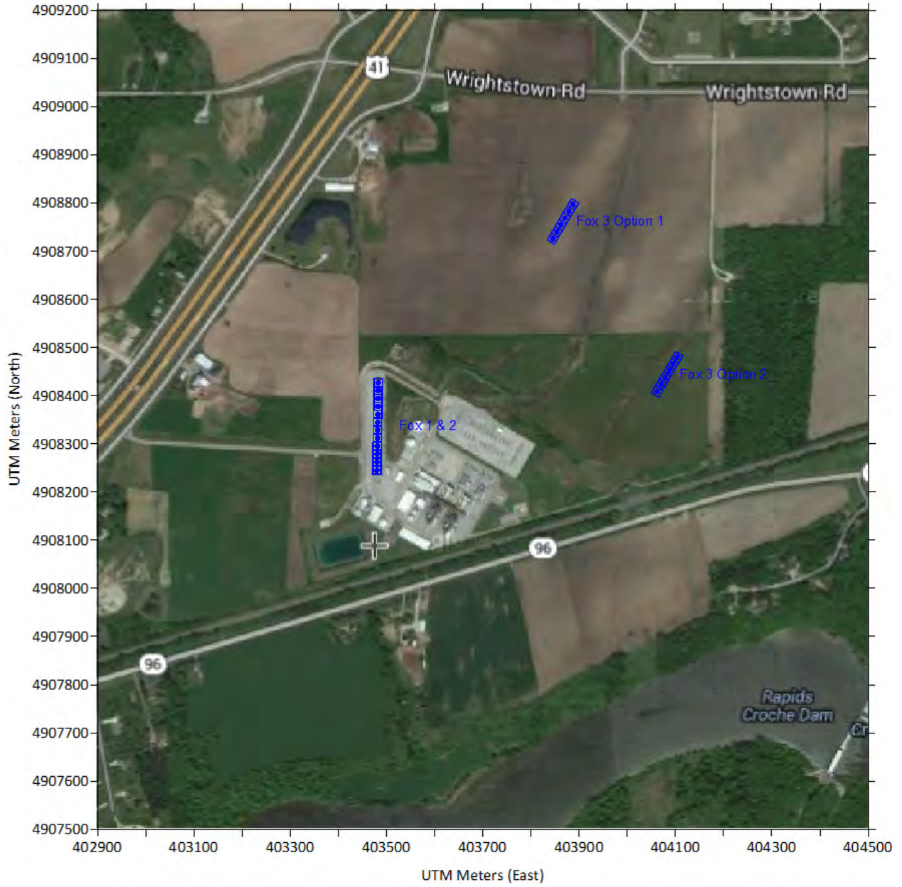
Figure 1: Fox 1 & 2 and Fox 3 – Cooling Tower Evaluation Locations
