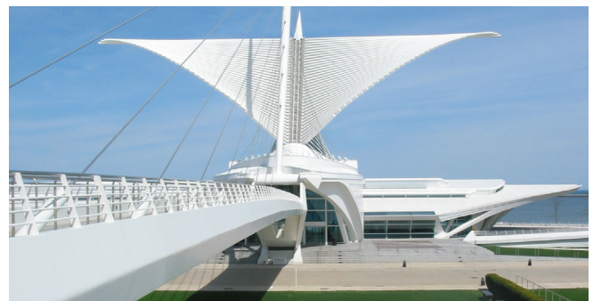
The Quadracci Pavilion at the Milwaukee Art Museum was constructed using We Energies fly ash.
